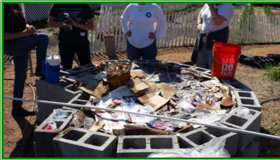
Ready for Top Soil
